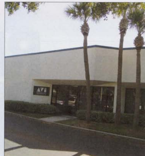
Founded in 1979 in Lakeland, FL, AVI set up its corporate headquarters (shown above) in 1981 in Tampa.
